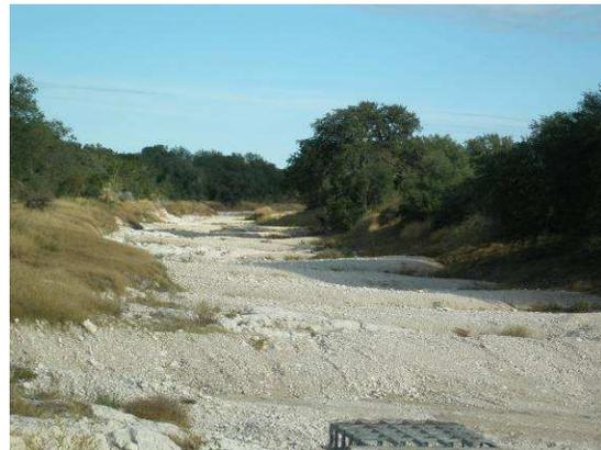
The tour took us to the sinkhole. They dug a canal so that stormwater runs directly into the ground and there are recharge holes where the channel flows water to the aquifer.
