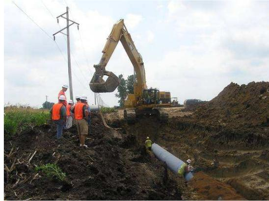
Some of the pipe further south near two planned 7.5 million gallon reservoirs will involve 54” inch pipe. In addition to excavation and pipe installation, the group observed the shrink wrap activity involved in sealing pipes together. On a good day, the workers can put in about 800 ft of pipe.
